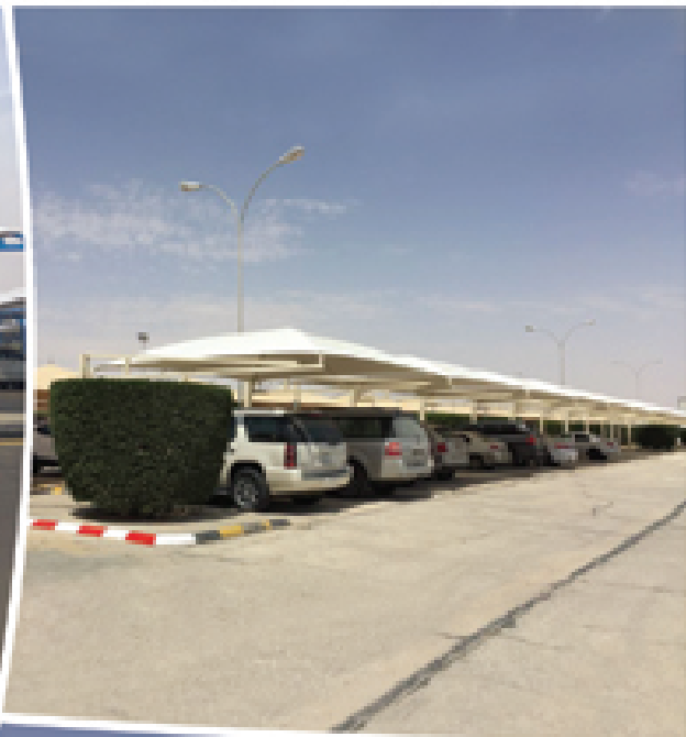
AL-HASAA AIRPORT Area : 6000 m 2 Year : 2016 Location : Al Hasaa Material : PVC
