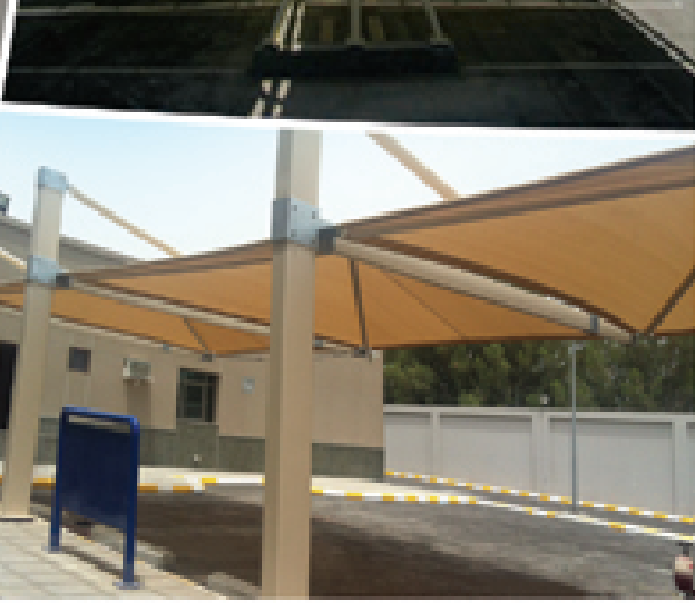
King Abdullah Project (KAP0) Patrol Car Shades Area : 20385 m 2 Year : 2013-2014 Location : Different Sites Material : HDPE
