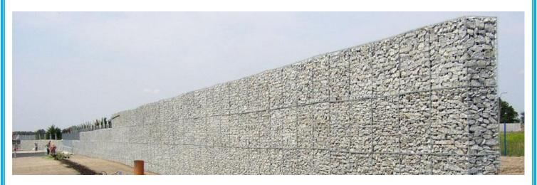
Gabions are rectangular wire mesh baskets filled with rock at the project site to form flexible, permeable, monolithic structures such as retaining walls for commercial, industrial and road projects. They are also used for erosion control, bank stabilization, channel linings and weirs.
